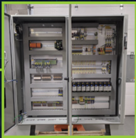
An overhauled production conveyor control system in under 4 months
